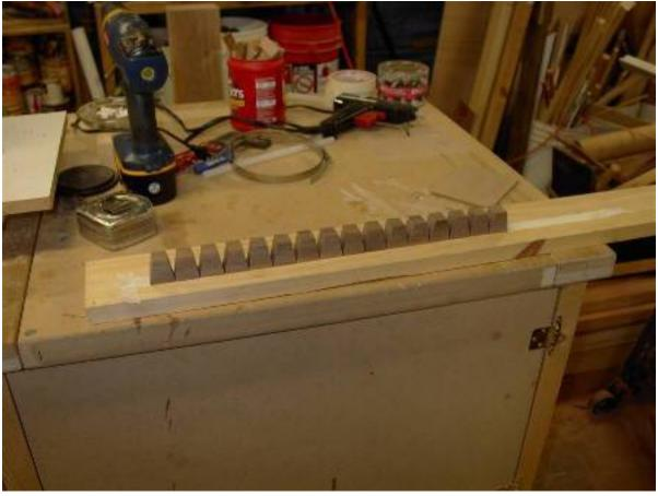
Apply glue to all mating surfaces and spread with a putty knife.
